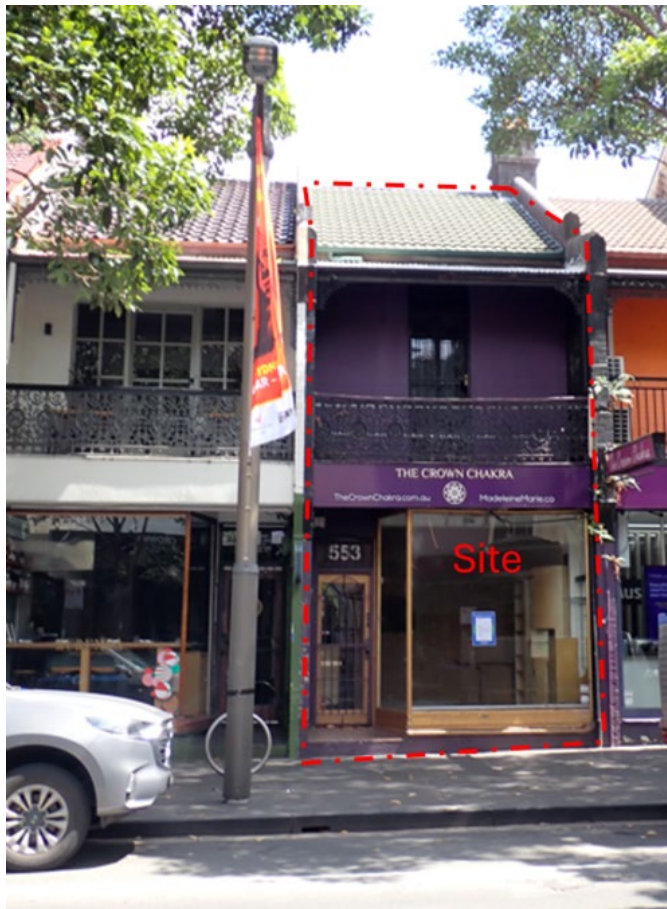
Site viewed from Crown Street
